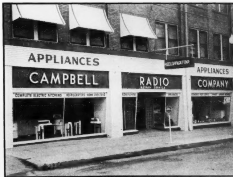
A MODERN BRICK BUILDING houses the Campbell Radio & Appliance Co. Slanted display windows eliminate glare and attract shoppers.
